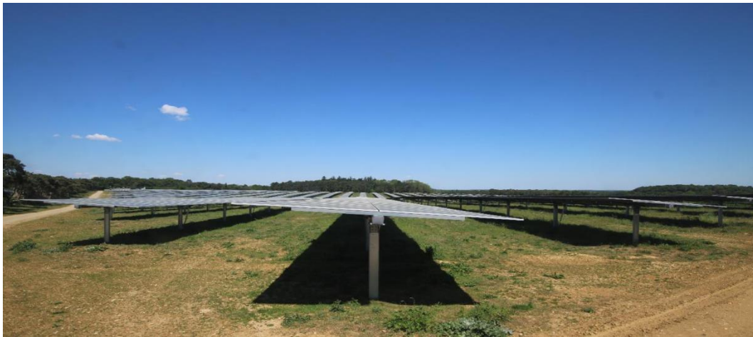
Plate 2-3 Illustration Tracker Solar PV Panels following the sun's positions
