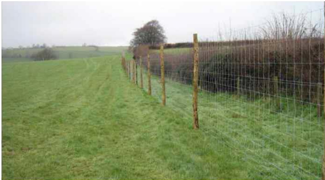
Plate 2-11 Typical Deer Fencing
