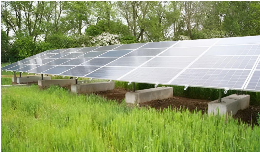
Plate 2-5 Fixed Panels on Concrete Feet
