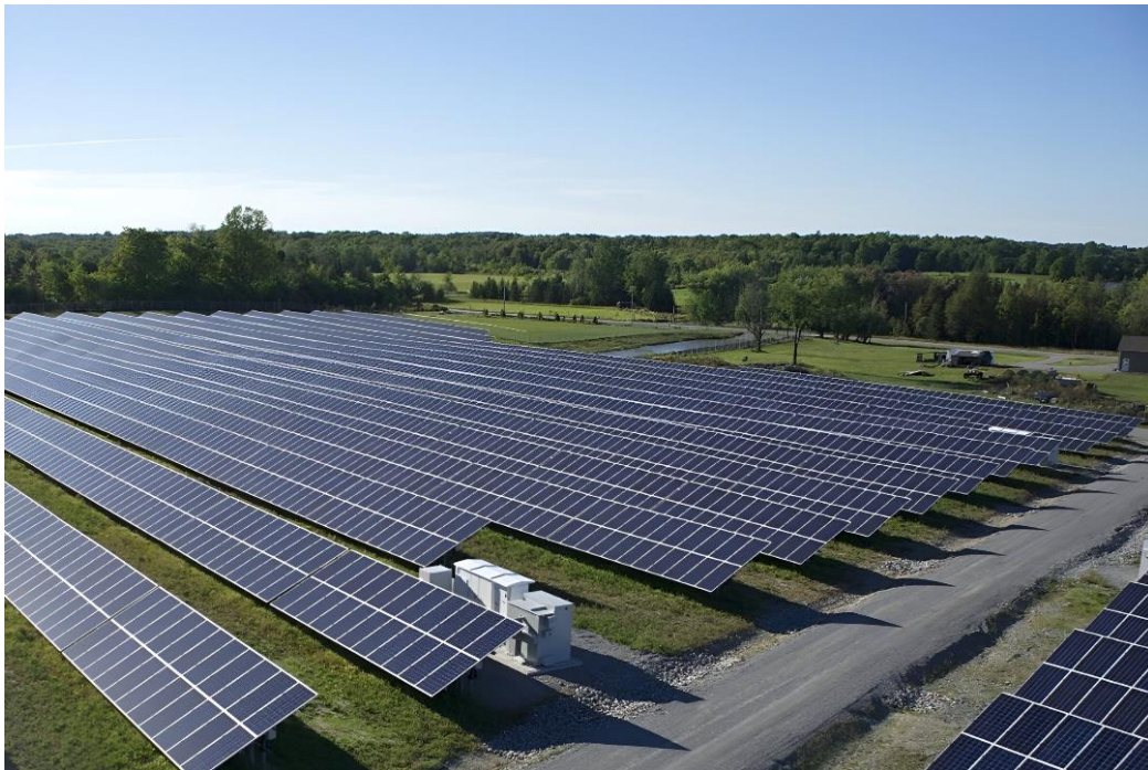
Plate 2-5 Fixed Panels on Concrete Feet
